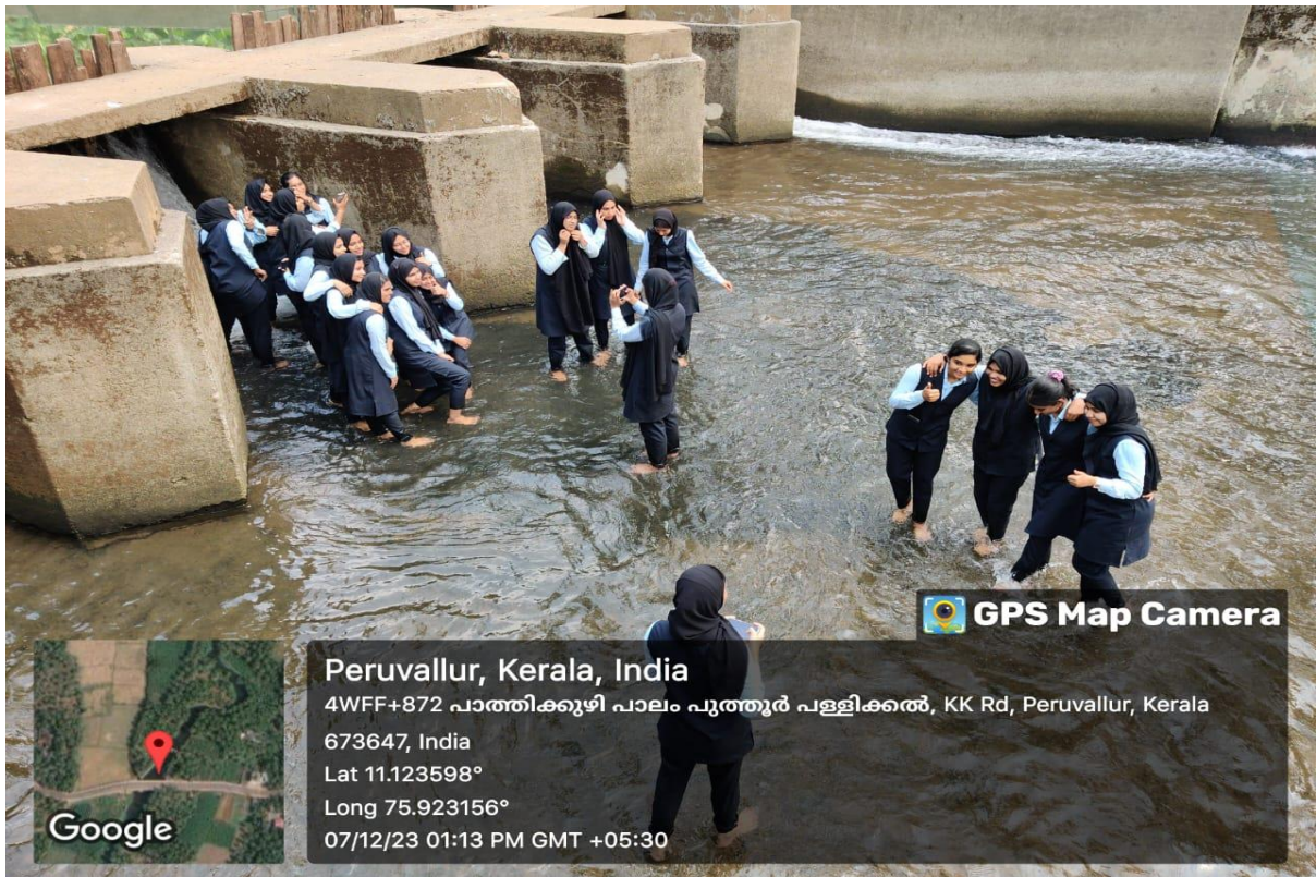
Pathikuzhi Check Dam one of the major sources of water of paddy fields in Pallikkal and Peruvallur Villages
