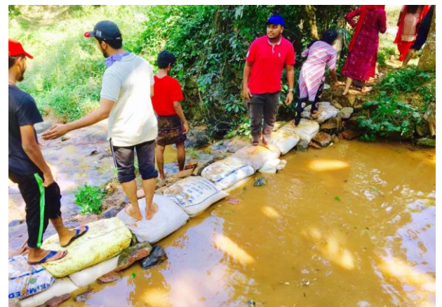
Check Dam Construction
