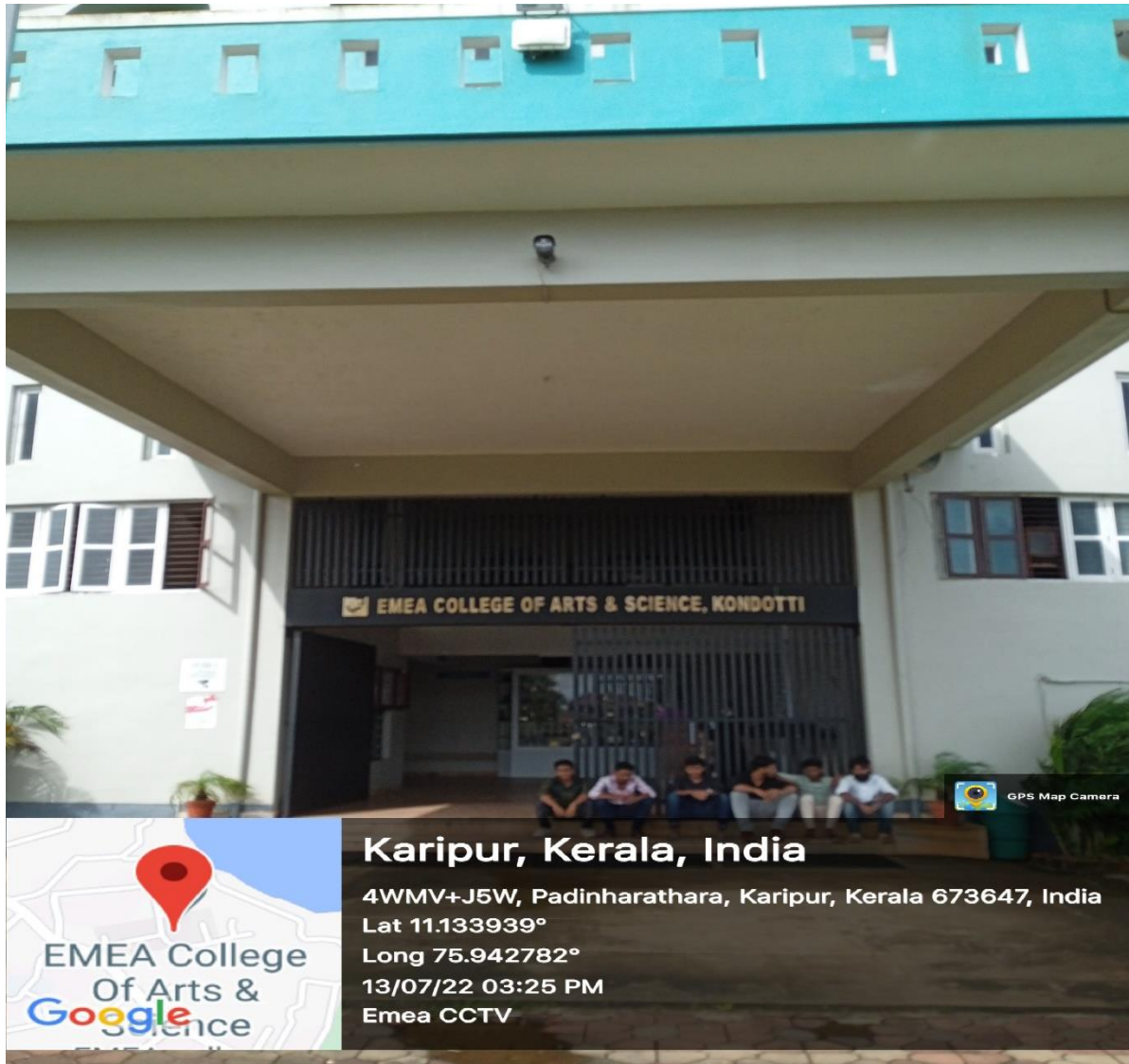
CCTV Camera at Main Entrance
