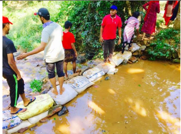
Check Dam Construction
