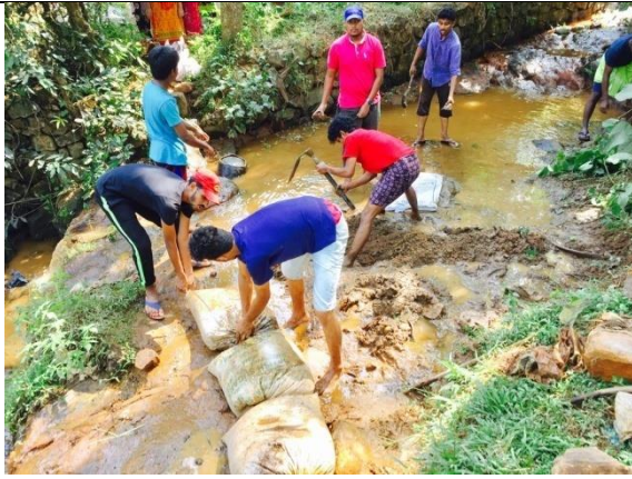
Check Dam Construction
